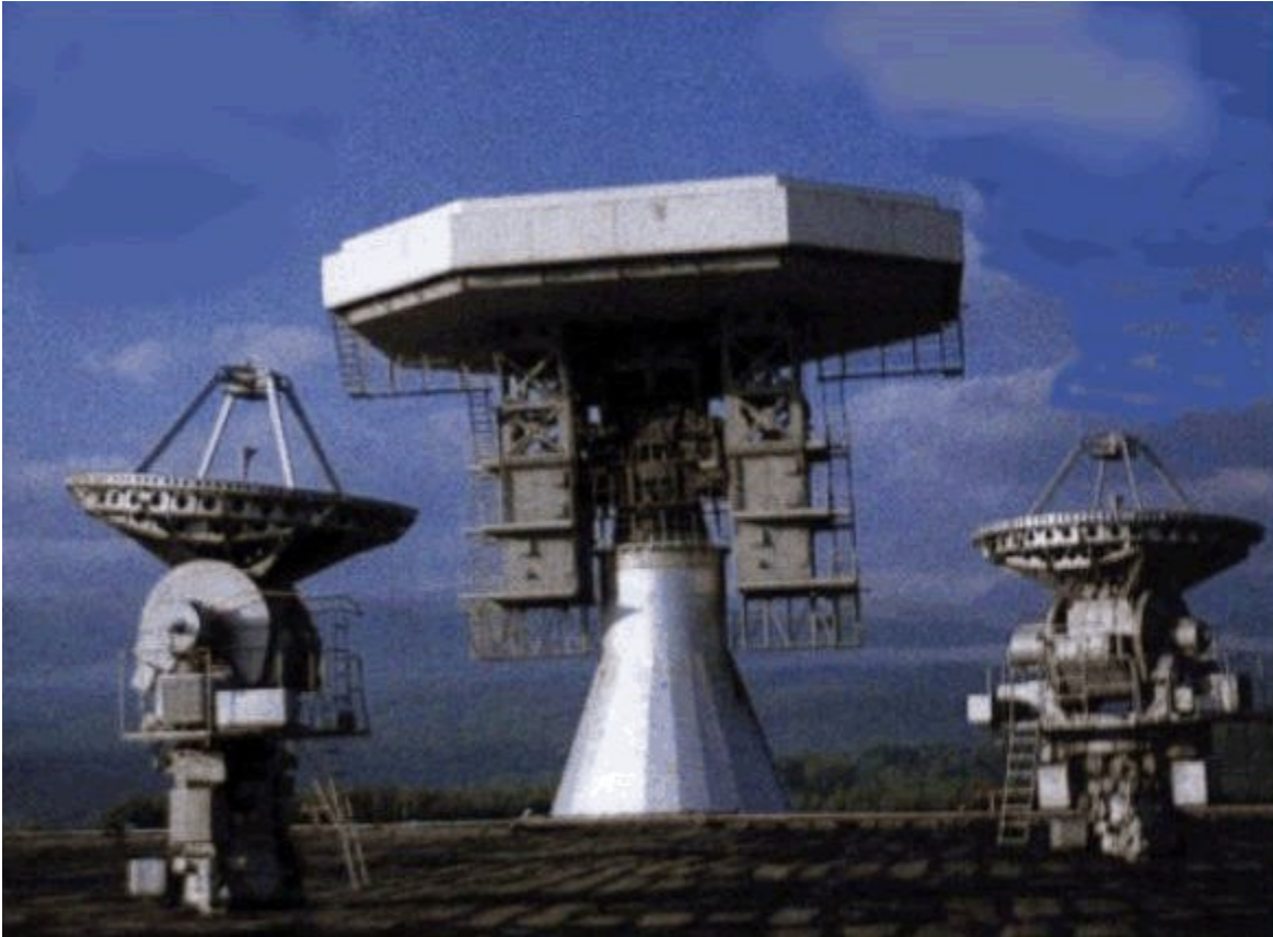
Krona Radar tracking and imaging facility
